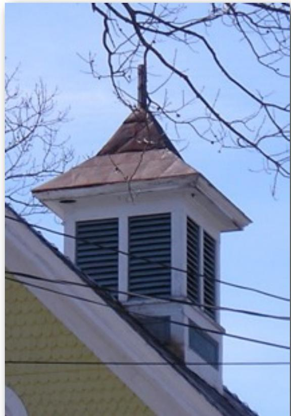
Paired rectangular shutters and paneled base. Wide hipped bonnet metal clad roof with carved post. While simple the shutters and panels contrasting colors compliment and enhance the overall carriage house design. Northern Maine, 19th century.
