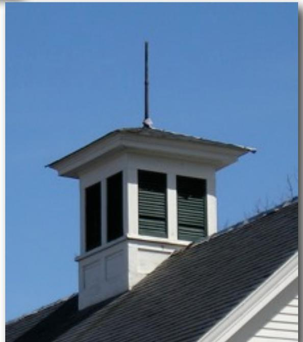
Another wonderful example of 19th century cupola design. Perfectly scaled and integrated into the carriage house's pavilion hip roof. A tapered cedar shingled base, paired arched shutters with proportionately spaced and sized louvers, moderately curved hip roof, finely detailed dentil, scroll and trim work. Notice the deep, steeply pitched sill. Contemporary weathervane. Western Maine, 19th century.
