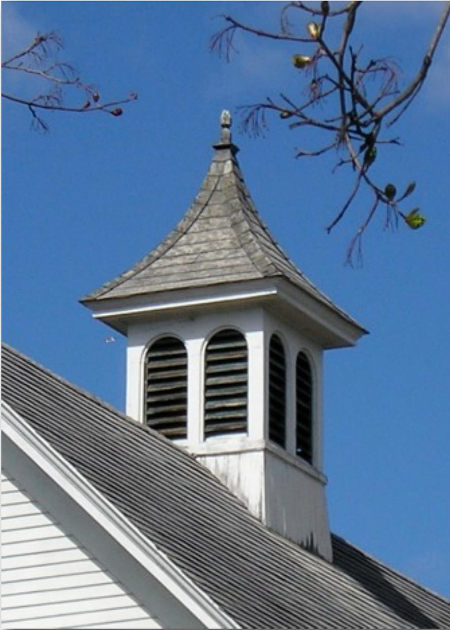
A beautifully balanced cupola. Almost oriental with its spare aesthetic. Wide high curving hip roof, tapered base with vertical tongue and groove face boards, simple paired arched shutters and trim work, and carved post. Notice the size and spacing of the shutter's louvers compared to the cupola's shutters below. Western Maine, 19th century. Approximately 4' x 4' x 8'-9"
