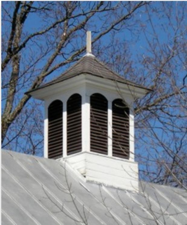
Simple but well proportioned. Large paired arched shutters, narrow columns, slightly tapered base with horizontal clapboards, and wide moderately curving hip roof with carved post. Western Maine, 19th century.
