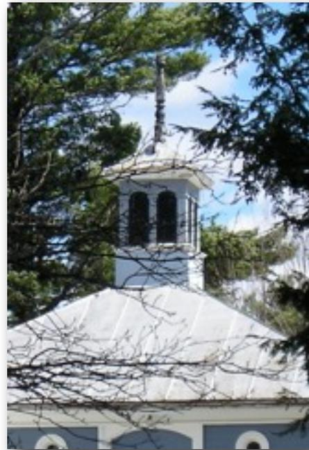
Nicely proportioned cupola with a massive turned post. Paired arched shutters and metal clad hip roof. Notice the unusual height of the cupola's base relative to the carriage house roof line. Kennebec river valley, Maine 19th century.
